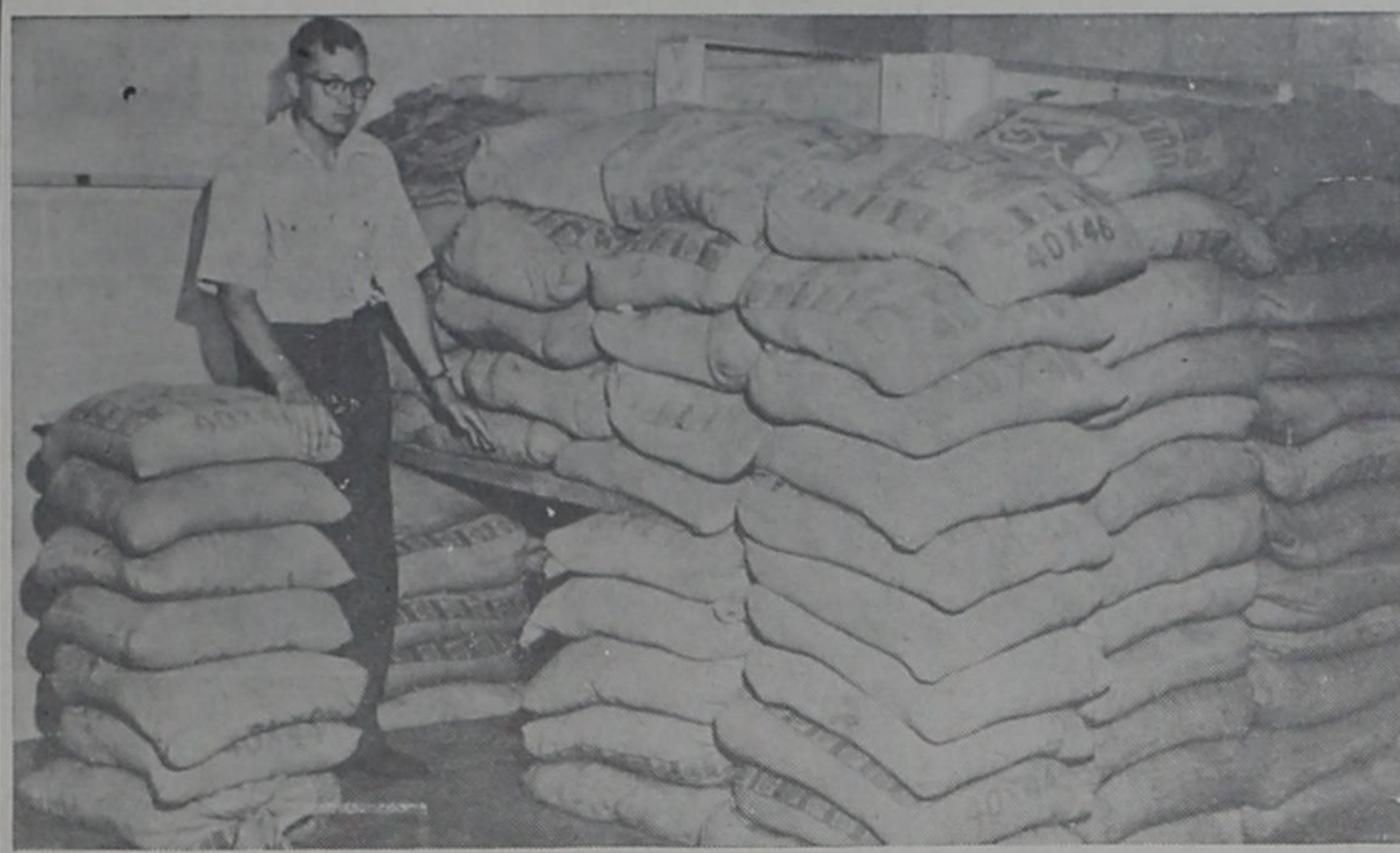
SANDBAGS FOR SAFETY —The nuclear scientist who designed this "poorman's fallout shelter," says that it will provide protection from fallout. The $30 dwelling, which was modeled after a British World War II shelter, had its first showing in Storrs, Conn.
