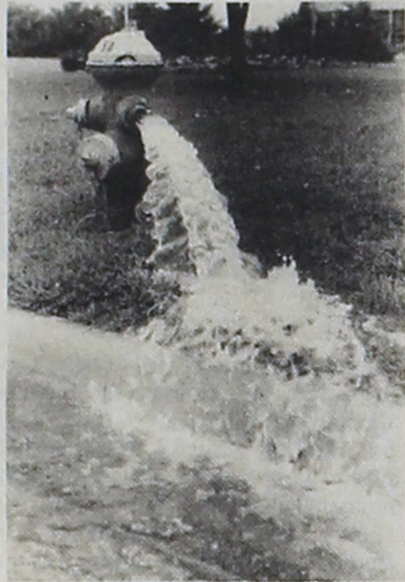
DAVID DITTFURTH, city employee, works on installing a new water line to Fischer's Meat Market earlier this week. The work on Second Street left some areas of town without water for a short time. At left, water is drained before the new line was put in.
