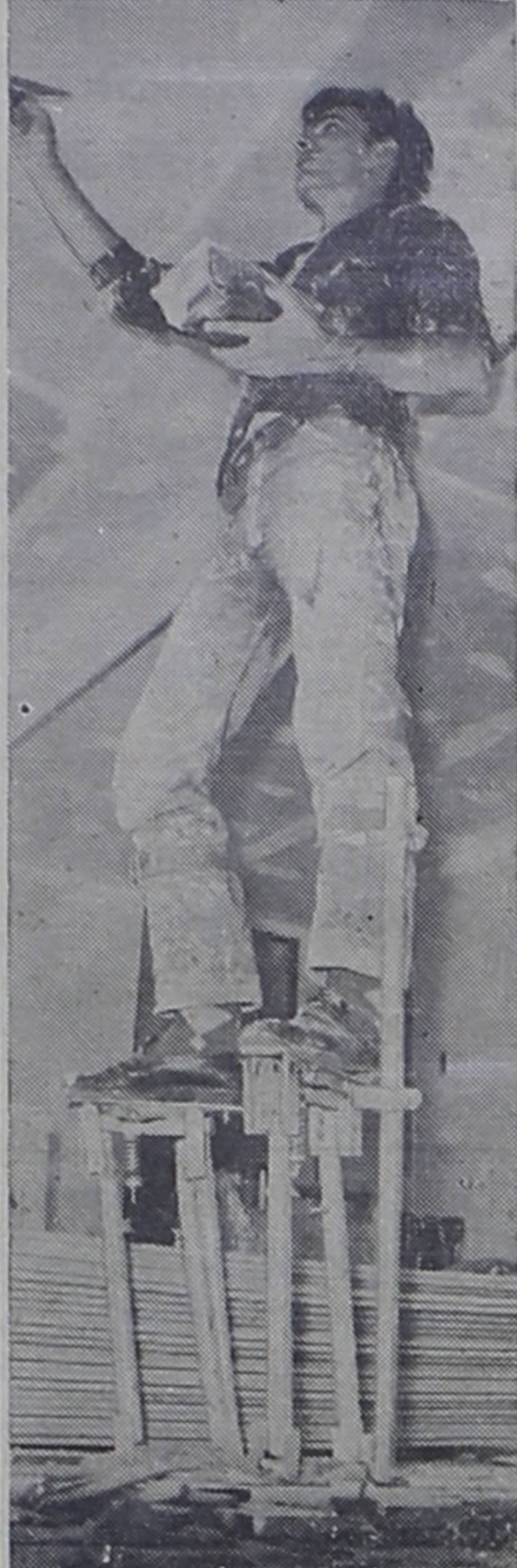
STILTED —Fred Berry says that using stilts helps him to reach the ceiling better than scaffolding for touch-up jobs he gets in Riverdale, Md.
