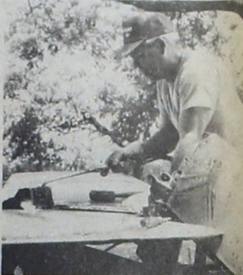
Dismantling was delayed when frozen bolts holding the tail wings couldn't be loosened. Above, David Fisher assists in the detaching; at right, Gilpin removes pins that hold the front and back fuselage (the body of the plane) together.
