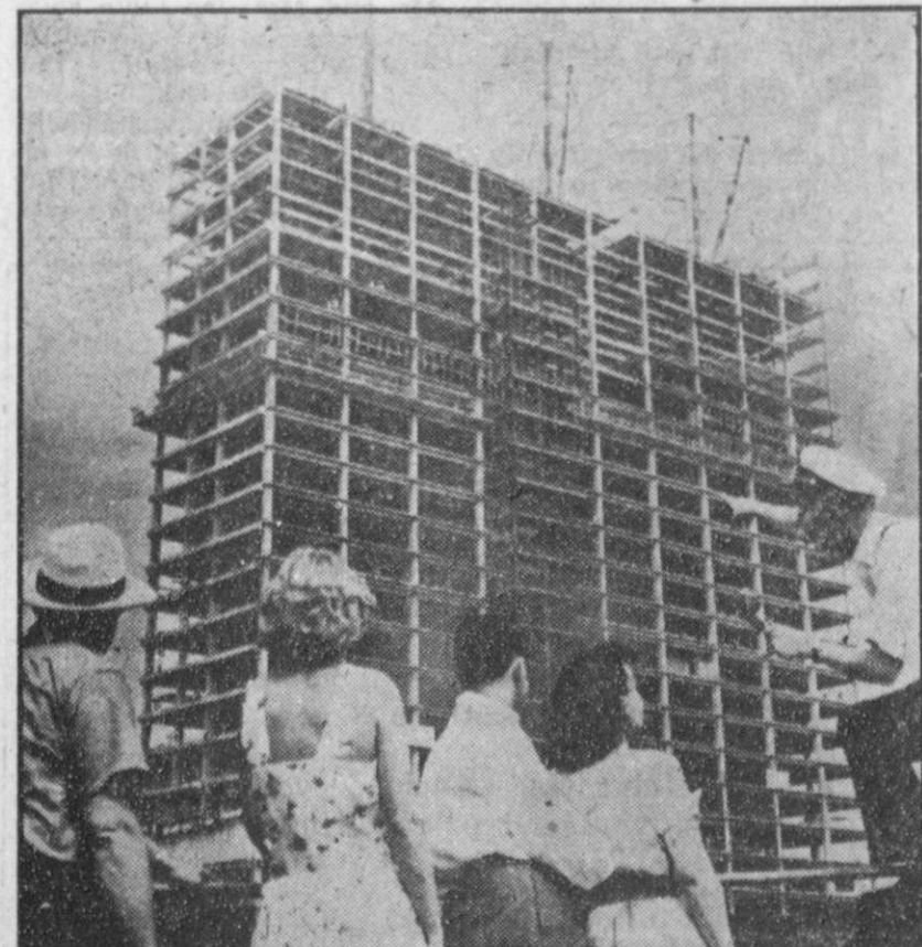
FRAMEWORK OF PEACE —Onlookers gaze at the progress being made on the new United Nations location in New York City. In the background is the skeleton of the U. N. Secretariat building, the first and tallest on the site. This 39-story structure will have 2700 air-conditioned offices.
