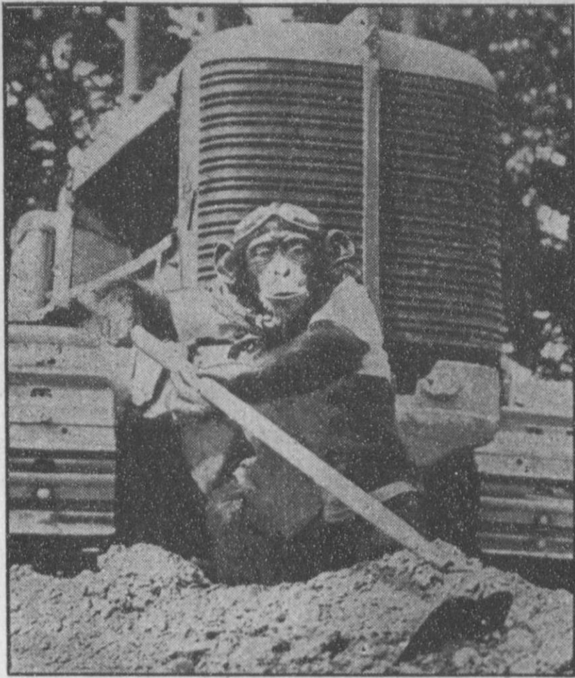
WILLING HELPER — This friendly-looking Pandora Chimp, resident at the Philadelphia Zoo, clears the way for a giant bulldozer. The task is one of breaking ground for a new lion house at the zoo. If the chimp's doing more than his share, it's probably because he wants to make sure the lions are kept well within bounds.
