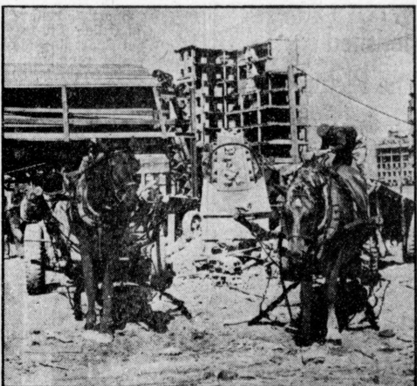
REBUILDING WARSAW —Rubble in war-torn Warsaw provides the bricks badly needed for the reconstruction of the city. Special mills, located near the devastated areas, are grinding and sorting the rubble for the concrete-mixing machines. The carts behind the horses are being loaded with rubble bound for the mill.
