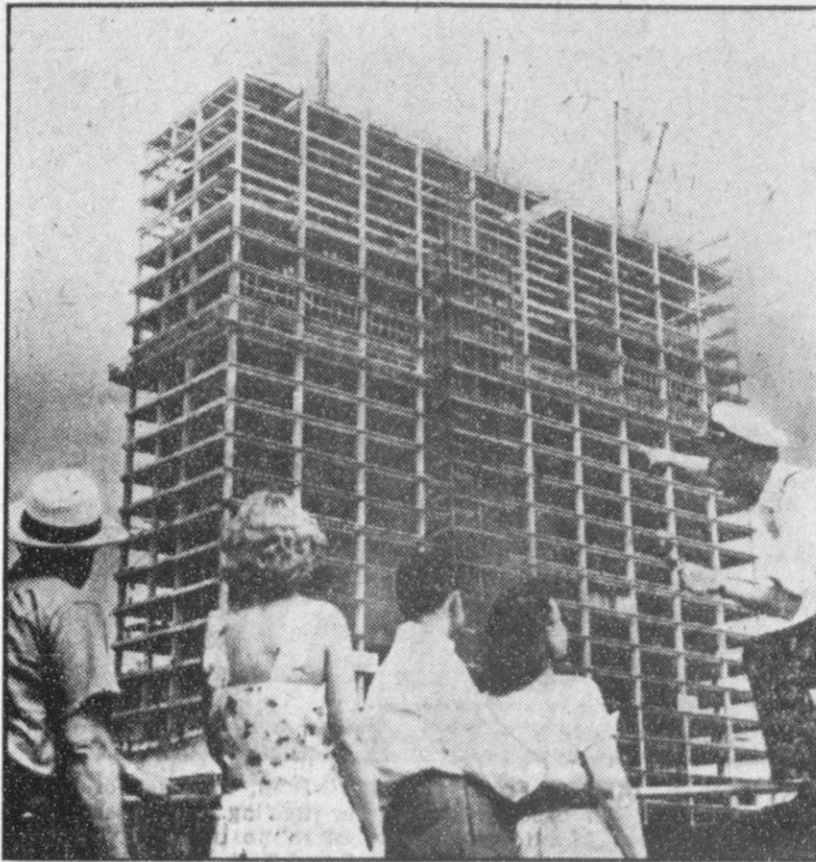
FRAMEWORK OF PEACE —Onlookers gaze at the progress being made on the new United Nations location in New York City. In the background is the skeleton of the U. N. Secretariat building, the first and tallest on the site. This 39-story structure will have 2700 air-conditioned offices.
