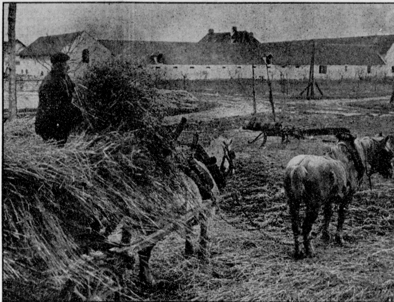
SITE FOR SHAPE —This quiet pastoral scene will soon become a beehive of activity as workmen move in to construct buildings for Supreme Headquarters, Allied Powers in Europe (SHAPE). Site is about 17 miles west of Paris and was personally selected by General Eisenhower, SHAPE's supreme commander. The tract takes in some 60 acres.
