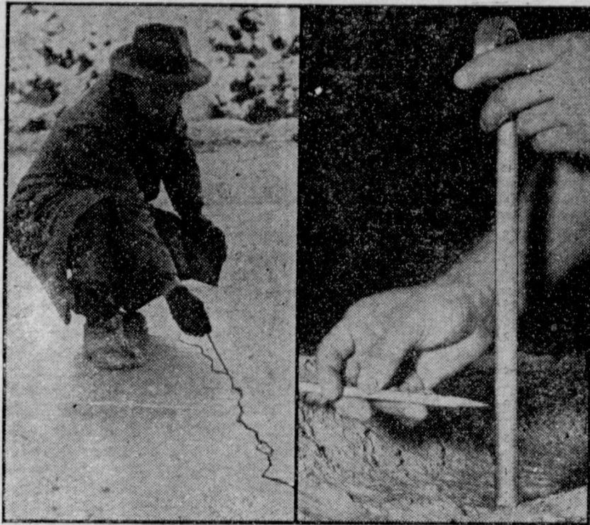
TEST ROAD FOR TRUCKS —U. S. highway engineers recently subjected a section of a heavily traveled state highway in Maryland to extensive tests in an effort to determine whether trucks damage the nation's roads. At left, an engineer measures a "typical crack pattern" caused by the multi-axled behemoths. After the equivalent of 98,000 trucks rumbled over the concrete test stretch, measurements (right) indicated the road had sunk almost three inches below its original level. As a result, highway officials recommended a maximum axle weight limit of 18,000 pounds for the cargo carriers.
