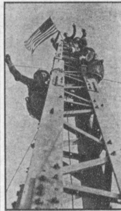
HIGH THERE! —Steelworkers, hanging from the highest point ever reached by a man-made structure, top off construction of the Empire State building's television tower with a flag-raising ceremony. The New York City skyscraper will now measure 1472 feet tall and accommodate five television antennas and three FM antennas.
