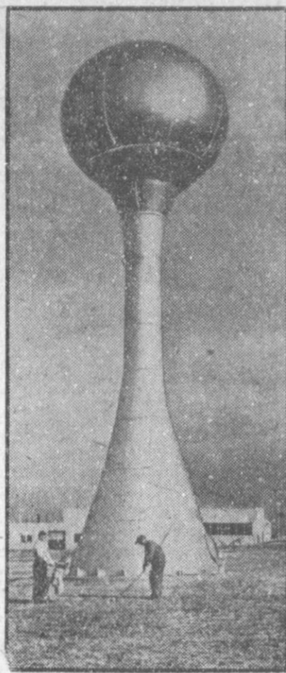
TEE-TOWER —This is not the golf tee and ball it appears to be at first glance. The oddly shaped structure is a water tower at the Shell Pipe Line Corp. pumping station in Cushing, Okla.
