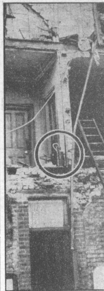
WRONG PROTECTION— Prudent owners of this house in West London, England, have kept their portable air-raid water pump (circled) ready for use all these years, but they never dreamed a freak wind-storm would slice off the side of their dwelling. No one was injured by the strange "twister" of fate.
