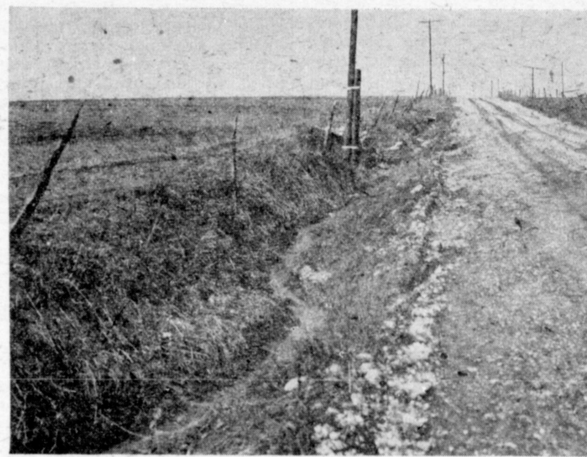
TERRACES EMPTYING INTO ROAD DITCH cause nothing but trouble and soil loss.
