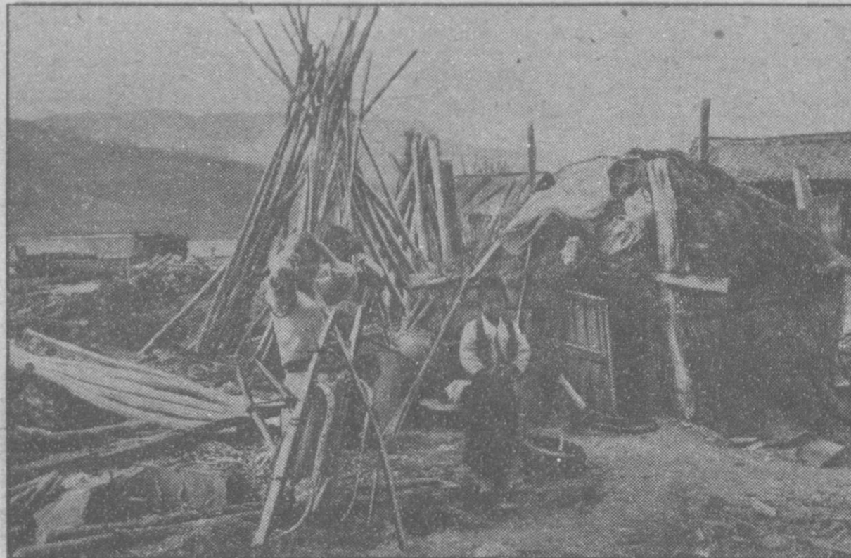
NEW ROOTS IN OIL SOIL—Using abandoned articles of war and stripped trunks of trees, South Korean refugees begin rebuilding in Yanggu, north of the 38th parallel. Some 100 families returned to the area, which they left before the Communist push south in June, 1950. While the main concern is constructing homes for their families, Korean men are beginning to till and plant the soil from which land mines have been removed.
