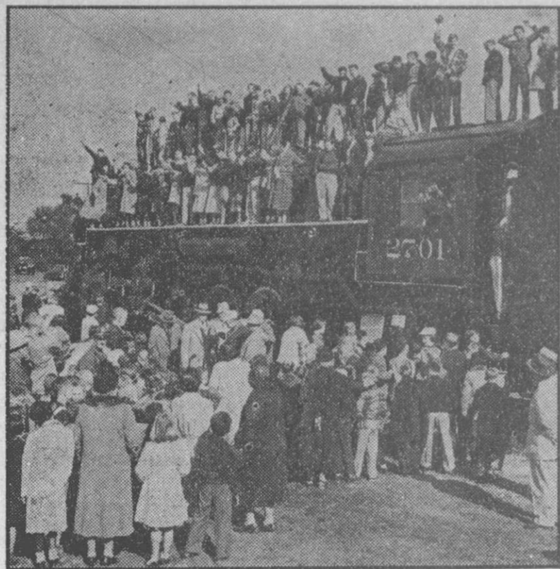
LOCOMOTIVE VALHALLA —Most steam locomotives considered obsolete go to the scrap foundry, but this Class K4 Kanawha high-speed freight hog has found a final resting place in La Salle Park, Buffalo, N. Y. Donated by the Chesapeake and Ohio as a monument to the age of steam which helped make Buffalo the nation's second largest rail center, it will be on permanent display for the enjoyment of oldsters and the amazement of a generation which is more familiar with the diesel locomotive. Built in 1943, the quarter-million-dollar locomotive is 105 feet long, weighs 425 tons with loaded tender and has pulled as many as 160 loaded coal gondolas at one time during its years of service.
