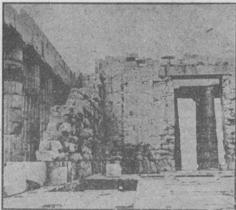
TEMPLE TO BE ROOFED—The Greek Archaeological Council will soon erect a roof over the ruins of the Parthenon, to protect the ancient Greek temple's sculpturing. The inner walls, such as the one shown to the right of the columns, will be demolished in hope of discovering ancient inscriptions of archaeological interest.
