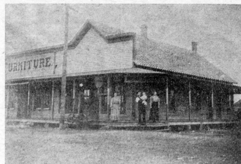
Taken in 1909, this picture shows the J. W. Meurers in front of his building which included his furniture store at the left his home at the right and the post office on the corner. The push cart, used to carry mail to and from the depot is in front of the post office. Mr. Meurer is holding his son, Herbert. One of the ladies is Mrs. Meurer, the other is Mrs. Susie Bernauer.
