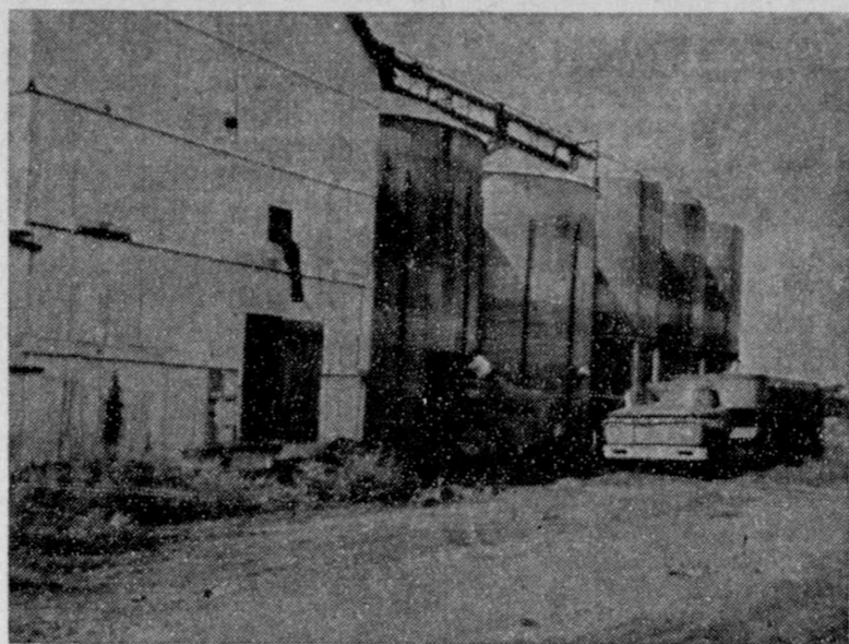
To clean up thousands of pounds of charred maize following last Friday's grain bin fire, Muenster Milling Company cut a hole in the bin large enough to admit a tractor with shovel. The fire is believed to have smoldered for several days before being discovered Friday and broke into flame after enough grain was removed to expose the glowing mass to air.
