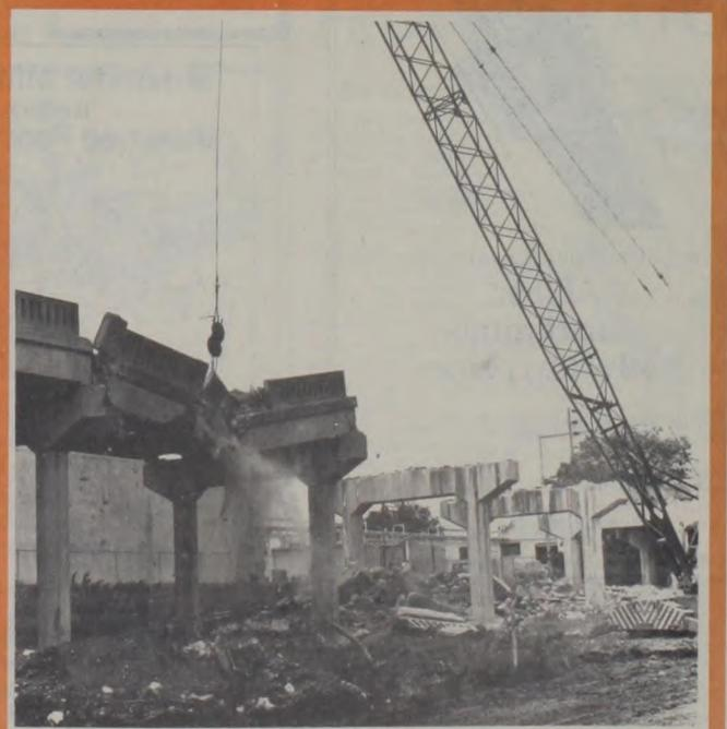
Going, Going, Gone! The Muenster overpass, shown here giving in to the impact of an 8000 pound wrecking ball, was demolished in less than three days. Wednesday night most of the supporting piers were still standing but the spans between were reduced to piles of chunk concrete and twisted reinforcing steel. --Photo by Art's Photos
