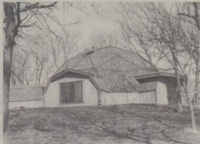
This Geodesic Dome Home, applying the principle of a sphere, is nearing completion for the Herman Carrolls north of Muenster. —Steve Luke Photo
