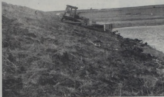
Picture 2 Bulldozer smoothing eroded area on dam. Three rows of common shoreline reedgrass and a strip of Alamo switchgrass are to be planted to aid in the control of wave action.
