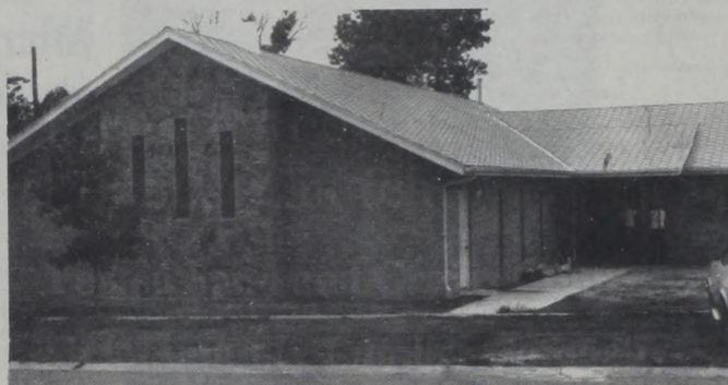
A large brick sign along with some landscaping will be done in the near future to complete the outside of the new church. Staff Photo
