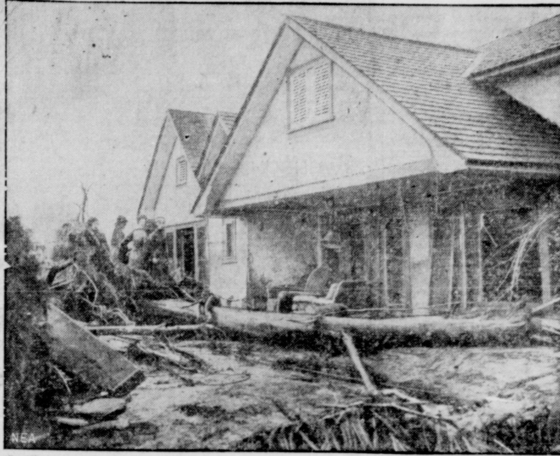
Struck by a wall of water, falling trees, and a huge mass of mud and boulders, this Glendale, Calif., home was wrecked by the storm and flood in Los Angeles county that killed 40 and caused $5,000,000 damage. Narrow escape of the family from death is shown graphically in the ruin wrought by the uprooted tree in front of the doorway and the mass of debris behind it.
