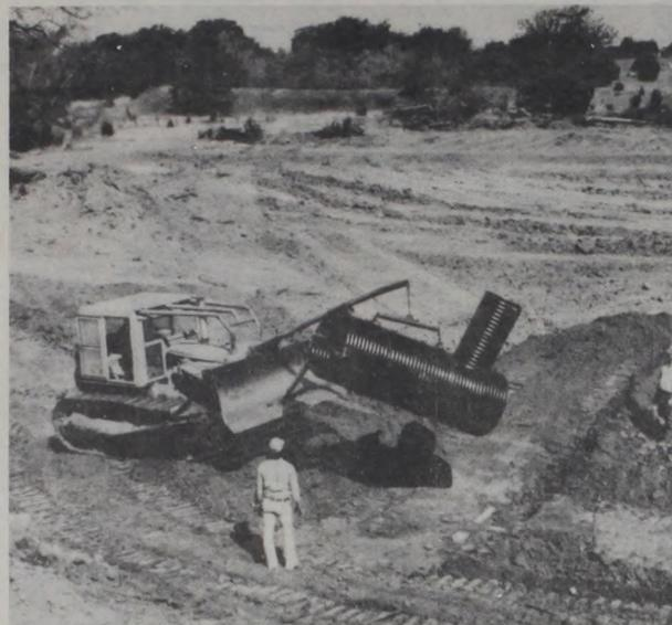
Grade stabilization structure being constructed to reduce erosion. SCS Photo
