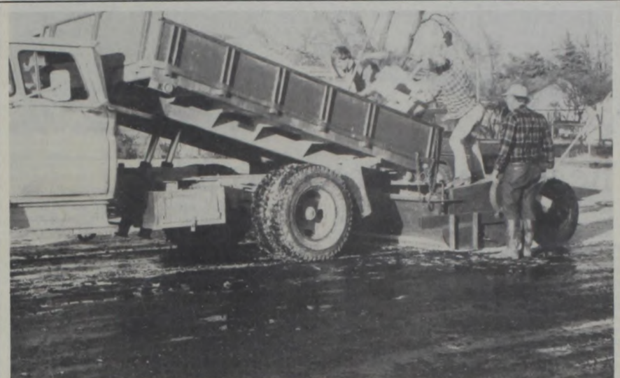
Muenster crews Tuesday afternoon were busy resurfacing some 660 feet of Second Street here, taking advantage of several paving projects planned within the city limits. Some down home ingenuity was displayed by the gravel spreader, a homemade engineering feat that was obviously working just fine.
