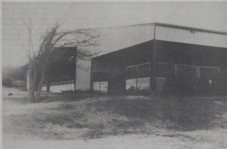
JAW Construction built this horse barn located near Rosston. Julian Walterscheid of JAW said there is probably 30,000 pounds of steel in the beams of the structure alone.
