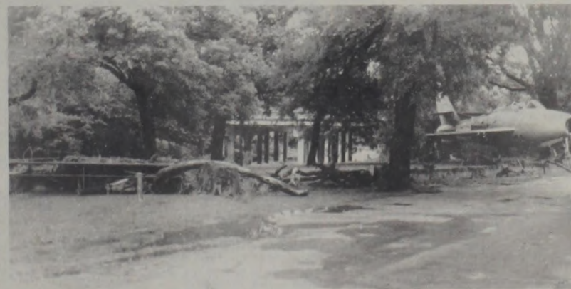
FLOOD DAMAGE WAS EVIDENT Thursday morning in the park as weeds, tree limbs, and in some cases whole trees were tangled along cables, wrapped around picnic tables, and cluttered the en-
