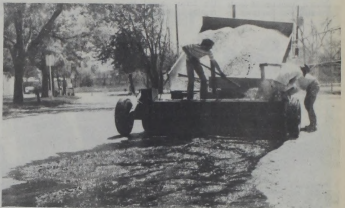
City crews have been busy repairing park roads.
