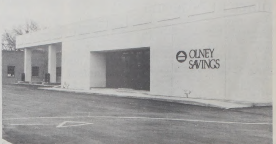
This front entrance of the handsome new Olney Savings Building at 1000 N. Grand in Gainesville will welcome visitors to the firm's grand opening of its Gainesville office on Saturday, the 7th 10 to 3. Olney Savings, originated in July 1927, has branch offices in 26 cities.
