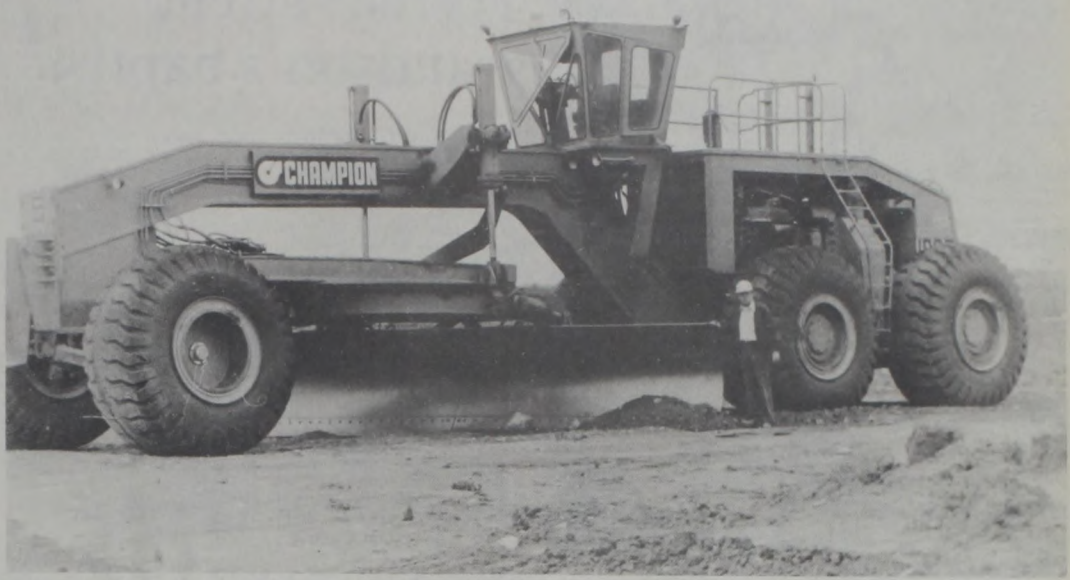
RESIDENT ENGINEER WEBSTER BOLAND is dwarfed by the huge grader being used to level dirt on top of the dam. The machine rents for
