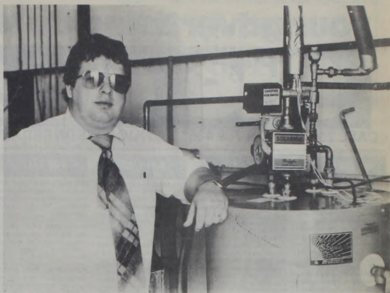
JIM WEEDN INSTALLS and services the water and home-heating systems Raypak builds.
