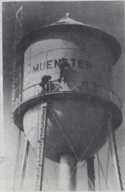
CREW WORKS on repainting the water tower. Janie Hartman Photo
