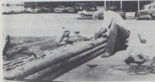
Doug Fleitman builds flower boxes on AMP1 lot.
