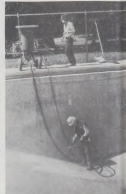
CITY CREWS sandblast the swimming pool, and add new paint before opening for the summer. Janie Hartman Photo
