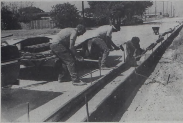
ENDRES ADDITION RESIDENTS can rest easier now as their long struggle to improve their neighborhood streets is bearing fruit. Charlie Knabe is setting curb and gutter forms on Mesquite Street. His
