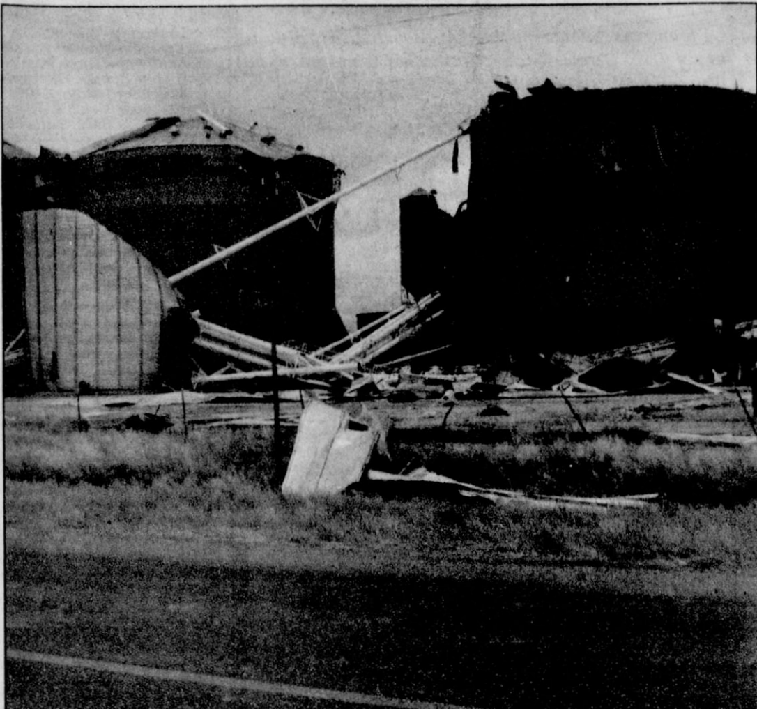
Pictured above is the AGCO Buzzard Elevator, located six miles south on FM 760, that was damaged in a storm on Thursday, June 5th. Photo by Gary Smith
