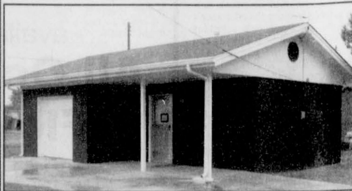
Pictured above is the newly renovated office for the Spearman Housing Authority.
