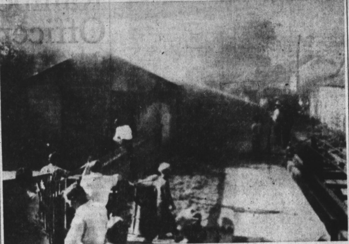
GARAGE BADLY DAMAGED by fire at 4:15 Wednesday afternoon was the property of Dan Finlin Second Street, flames were threatening a dwelling nearby fanned by a high wind when the Hereford Fire department arrived at the scene, and quick action on the part of the fireman prevented the spread of the blaze to the other property. The building was said to contain storage goods and some rubber tires, which accounted for the dense smoke, the blaze had possibly been smoldering for some time before it burst into flame, the cause or the damage was not known. Staff Photo.
