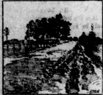
CONSTRUCTING A SAND-CLAY ROAD.
