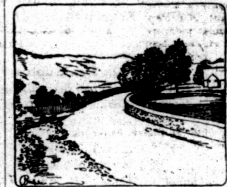
CURVED WALL AND ROADWAY WHERE A SIX FOOT FILL WAS MADE.
