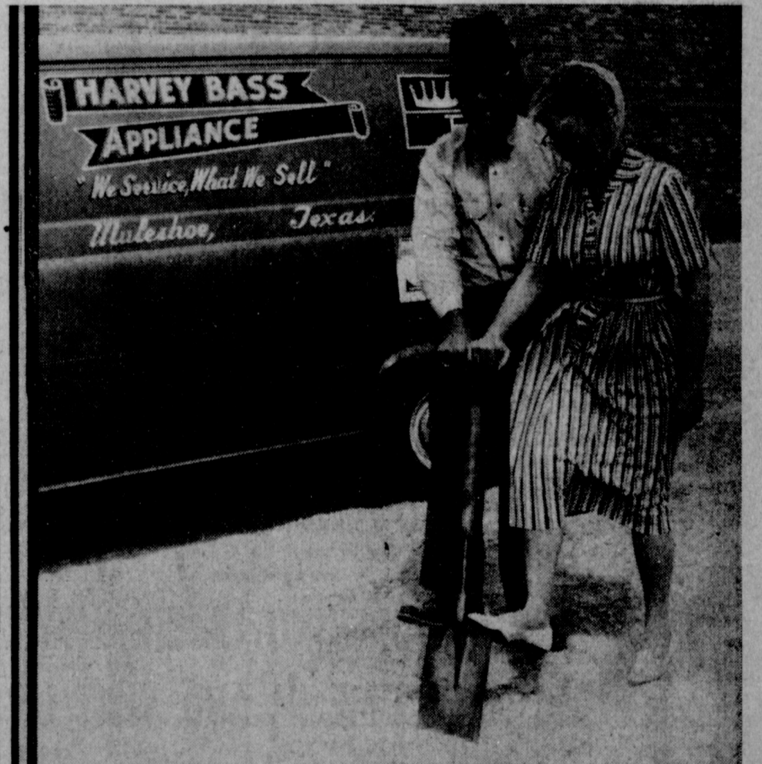
FIRST SHOVEL Mr. and Mrs. Harvey Bass moving the first shovelful of dirt to level the property upon which their new store will be erected. Costing about $50,000 the new structure, located across from Red's Super Market, is expected to be opened about the end of July or the first part of August. Bass said the new store will enable him to better serve his customers whose kindness and business has allowed the expansion.
