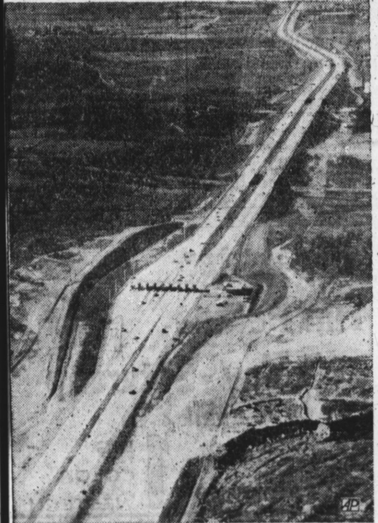
ADVANTAGE OF TURNPIKE—Fore plaza at Dallas end of Dallas-Fort Worth Turnpike illustrates convenience provided motorists for paying fares to ride the $58 1/2-million super-highway. More exit lanes than entrance lanes speeds up movement of traffic, and it's one of a total of two stops turnpike travelers make, compared with 45 traffic lights on U. S. Highway 80 and 19 on U. S. Highway 183. (AP Photo)
