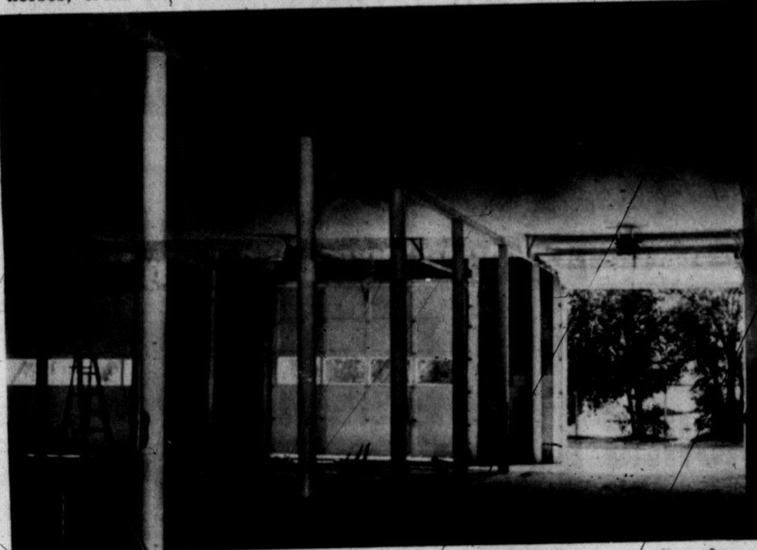
NEW QUARTERS — With the purchase of the building immediately south of City Hall, remodeling work has resulted in a new fire department building, which is almost complete.
