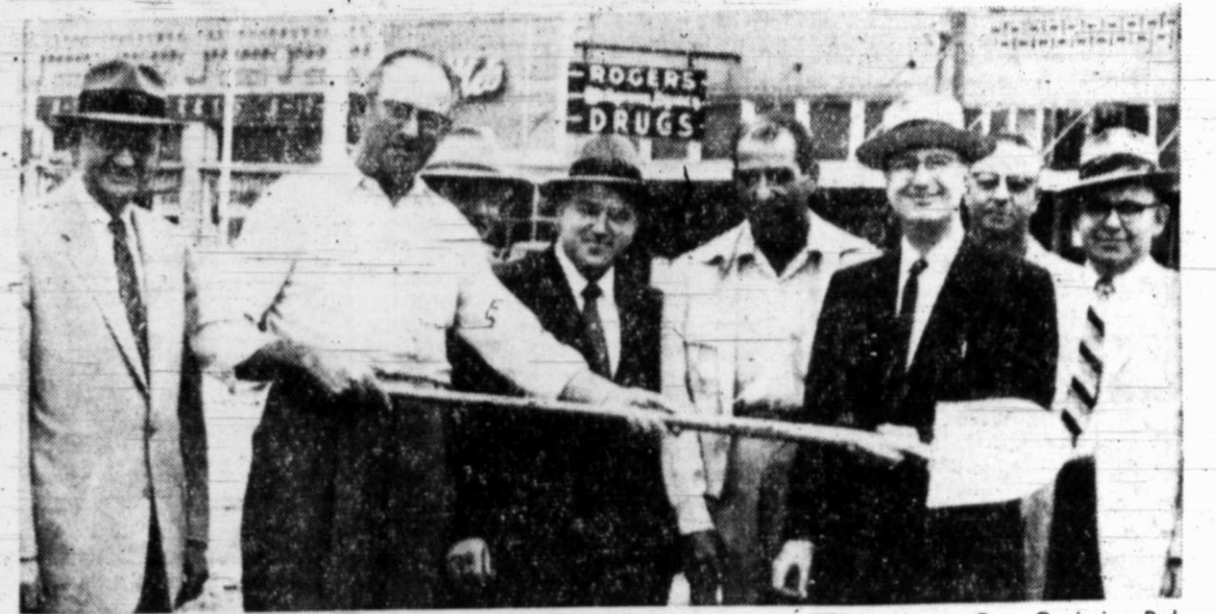
GROUND BREAKING—The first earth was turned to mark the start of construction Tuesday of a new $231,000 First National Bank building at Main and Third. Holding the silver shovel with which the start was signalled are J. A. Pitman, in shirtsleeves, and James Witherspoon, bank directors. Virgil Hennen, left, executive vice president; Virgil
