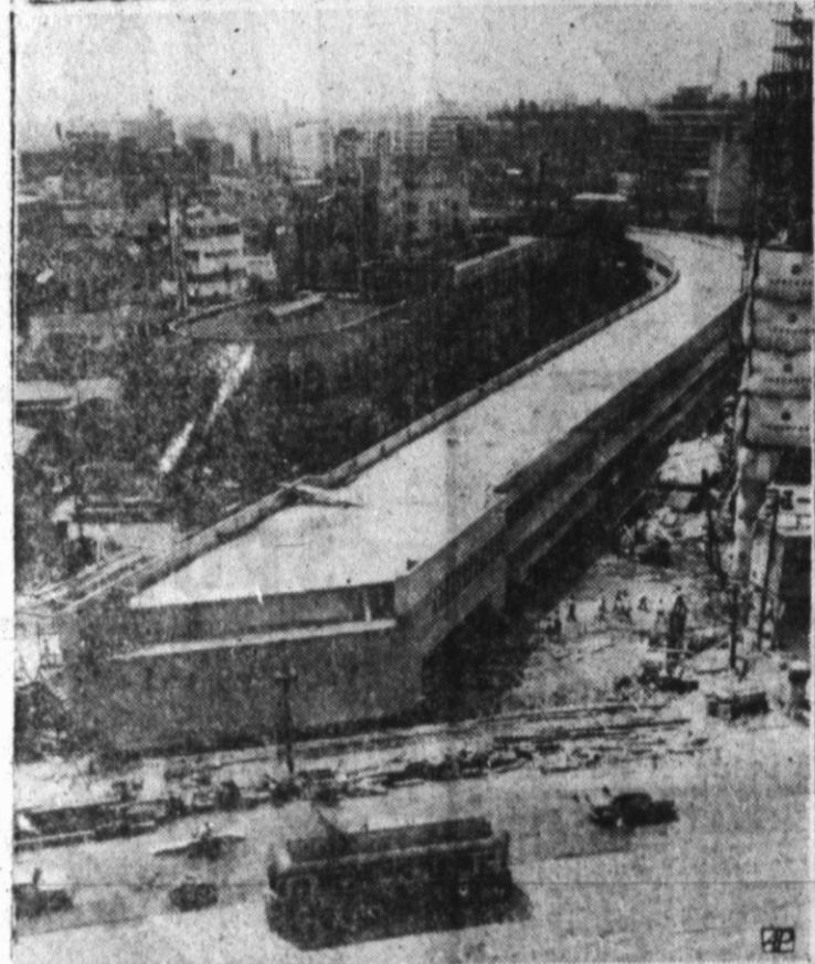
ROAD ABOVE, BUILDING BELOW—Here's a Japanese method for conquering city traffic problems—an expressway on the roof of a serpentine building. The roadway will not be complete until next year, but stores and tea shops already occupy parts of the building which winds through the heart of Tokyo.
