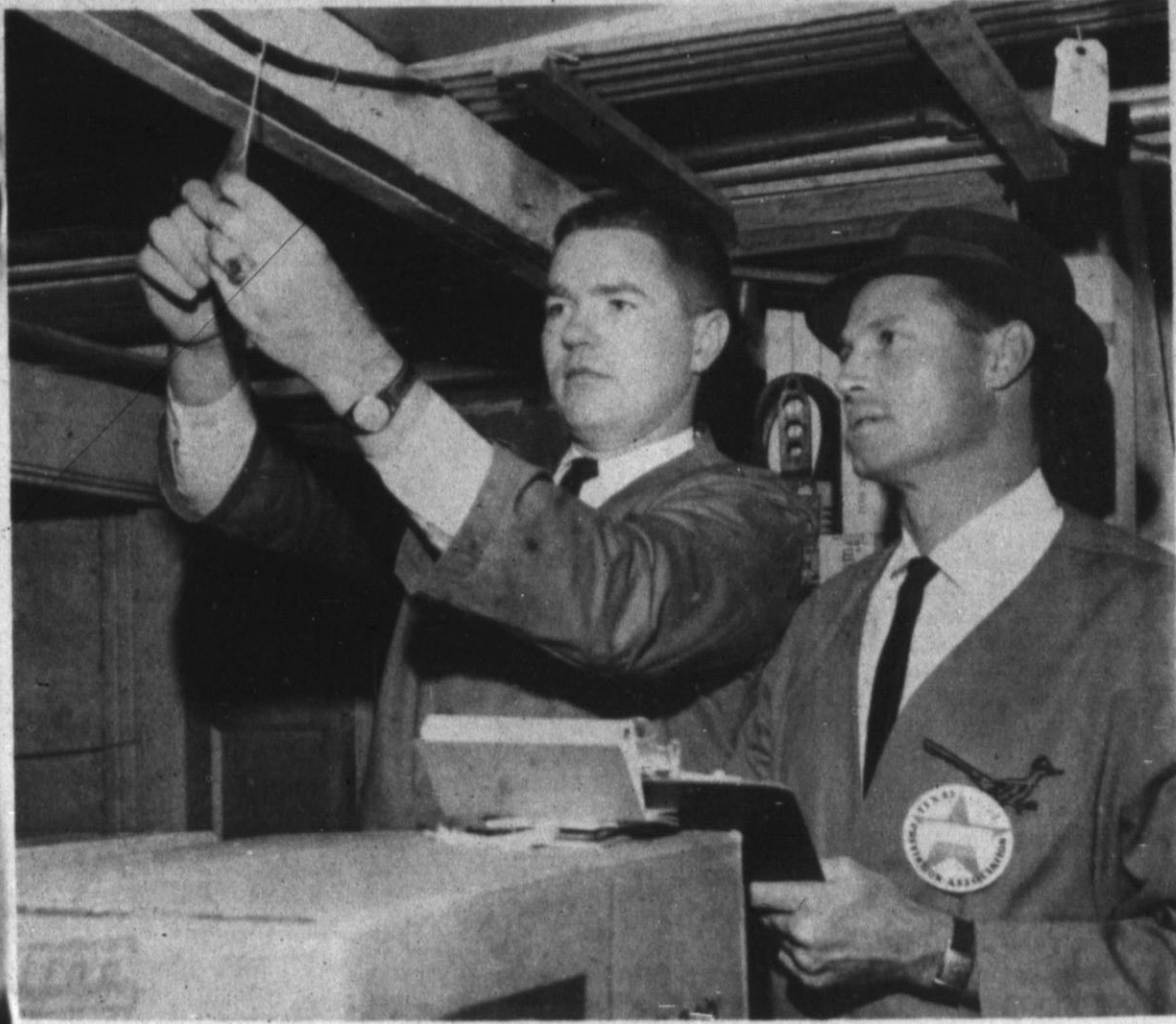
FIRE HAZARDS WERE red tagged as inspectors searched Hereford businesses, churches and schools during the voluntary inspection Wednesday. Inspectors Pat Boland, left, and Bob Moore tag one of the most common, an electric wire held in place by a nail. The inspection was sponsored by the Hereford Volunteer Fire Department as part of the Fire Prevention Week program. (Staff Photo)
