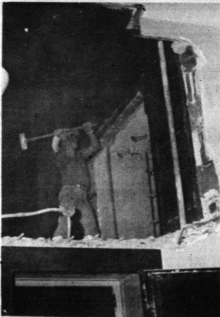
DEMOLITION — Crews had to tear out partitions, remove fixtures and postal windows to get the old post office building ready for remodeling. The haze in the picture is just plain dust that made a screen around workers. (Staff Photo)
