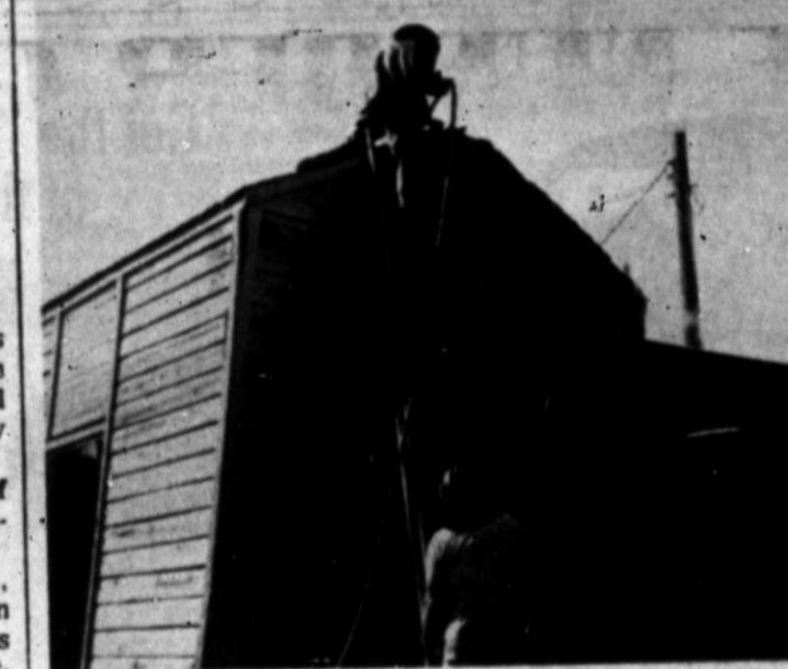
BURNED DOWN — This barn on the L. B. Wortham farm south and east of Hereford was hit twice by fire within three days, with the last fire Monday destroying it. Wiring caused a fire Saturday afternoon, when this photo was taken, but light damage was done that time as Hereford Volunteer Firemen had little difficulty putting it out. However, lightning reportedly struck the building shortly before 7 p. m. Monday and the building burned. Damage was estimated at $6500, with the greater portion of that amount being in tools which were stored in the barn.
