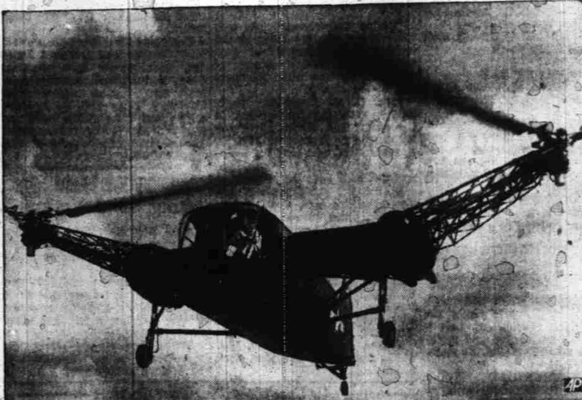
TWIN-ENGINE HELICOPTER —The U.S. Navy's XHJD-1, world's largest and first twin-engine helicopter, flies over Lambert-St. Louis, Mo., municipal airport in its first test. The twin engines give the plane greater reliability for safety over rough terrain, populated areas or water. The new machine will cruise at 100 m.p.h. with a load of 3,000 pounds.
