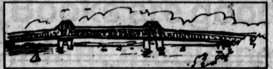
The longest cantilever bridge in the United States is the John Barry Bridge, in Chester, Pennsylvania. It spans the Delaware River and measures 1,644 feet.
