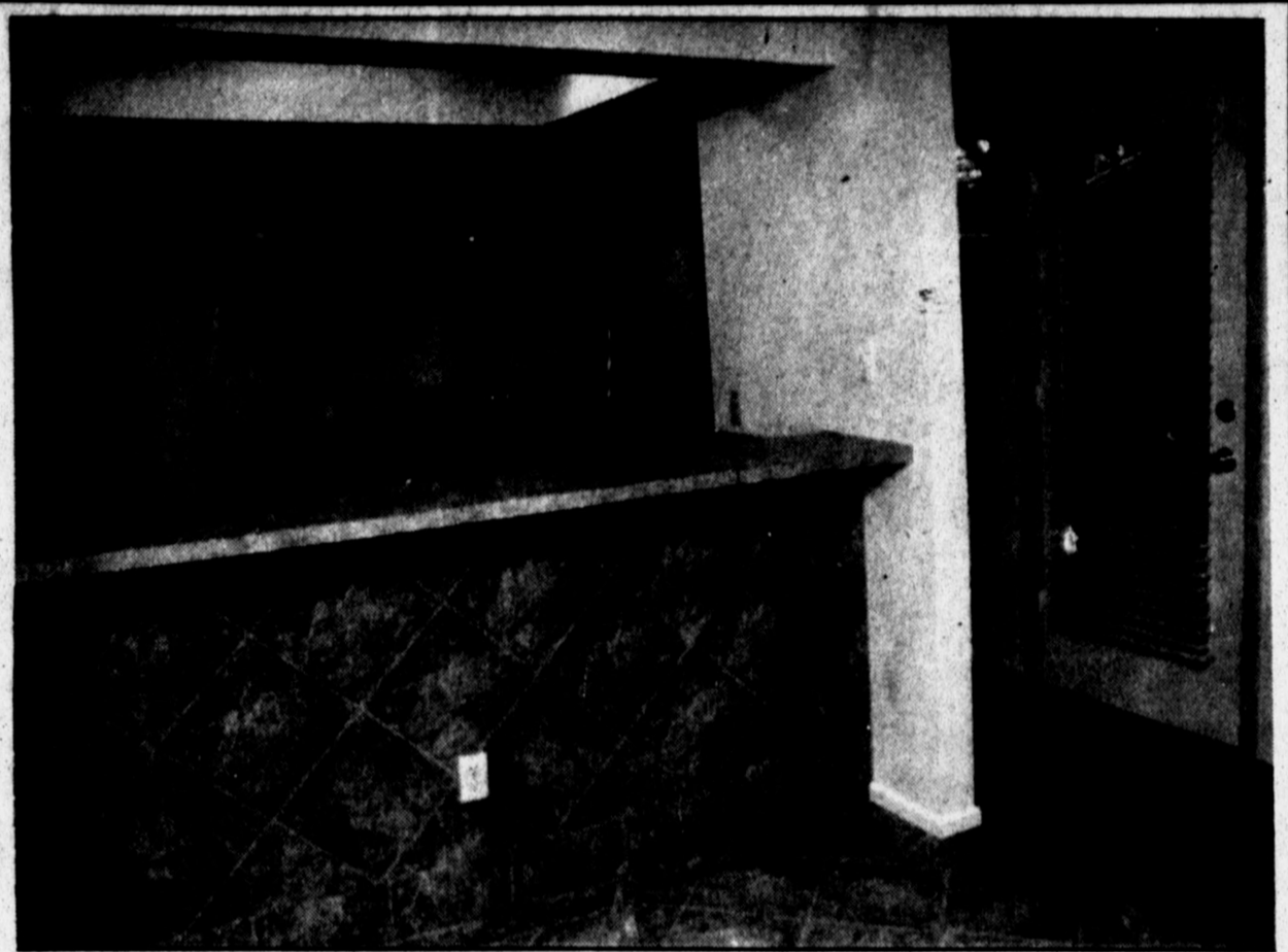
Quarry tile has been installed in the downstairs area of this apartment as part of an extensive remodeling project. Removing some cabinets and using track lighting have added much needed light to the small kitchen area as well.
